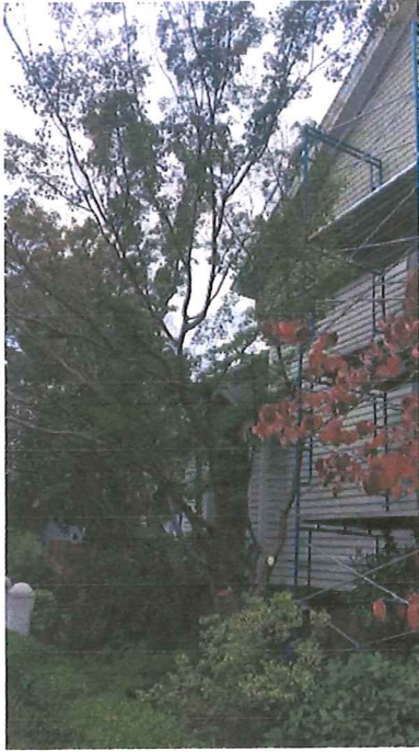
Tree 4 – Proximity to bldg
